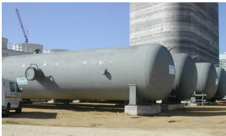
Figure 132: Steam accumulators at the PS10 Abengoa solar tower plant in Seville, Spain. (Reproduced from pole-derbi.com).
