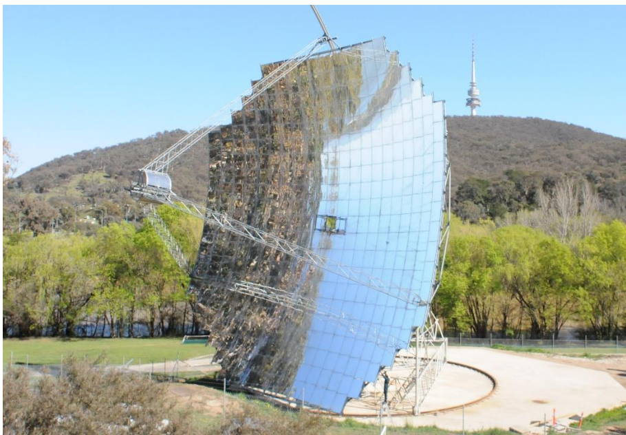
Figure 116: Australian National University's prototype 500 \text{ m}^2 paraboloidal dish concentrator (image K Lovegrove).
