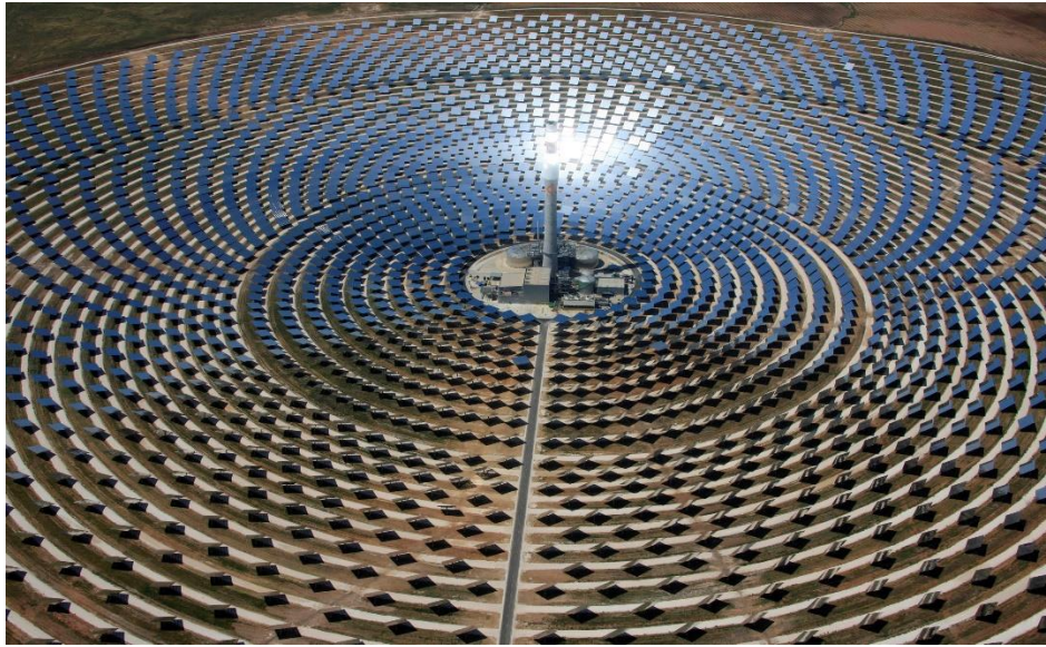
Figure 115: Aerial view of the Gemasolar solar tower plant in Spain, thermal capacity 400 \text{ MW}_{th} . (Image from Torresol Energy).
