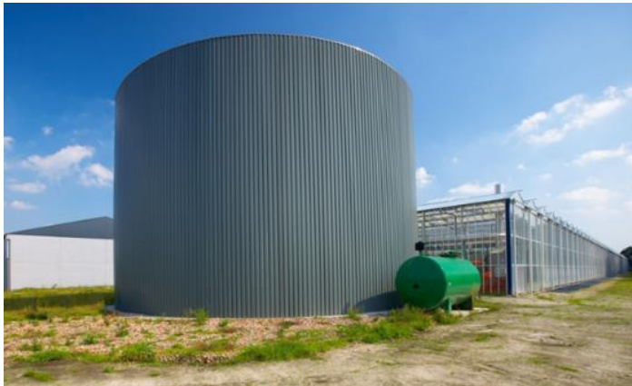
Figure 130: Unpressurized hot water storage tank operated between 65 and 85°C. (reproduced from Agricultural Projects Holland B.V.); right: pressurized storage tank. (Reproduced from I.VAR. Industry).
