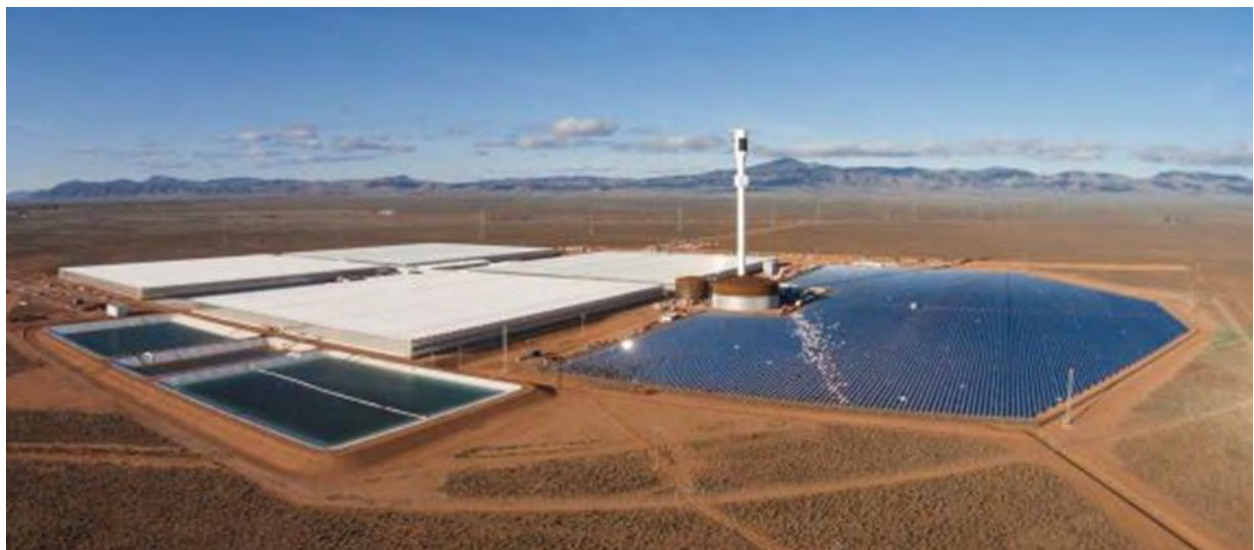
Figure 18: Sundrop Farms greenhouses and concentrating solar power plant (image Aalborg CSP).
