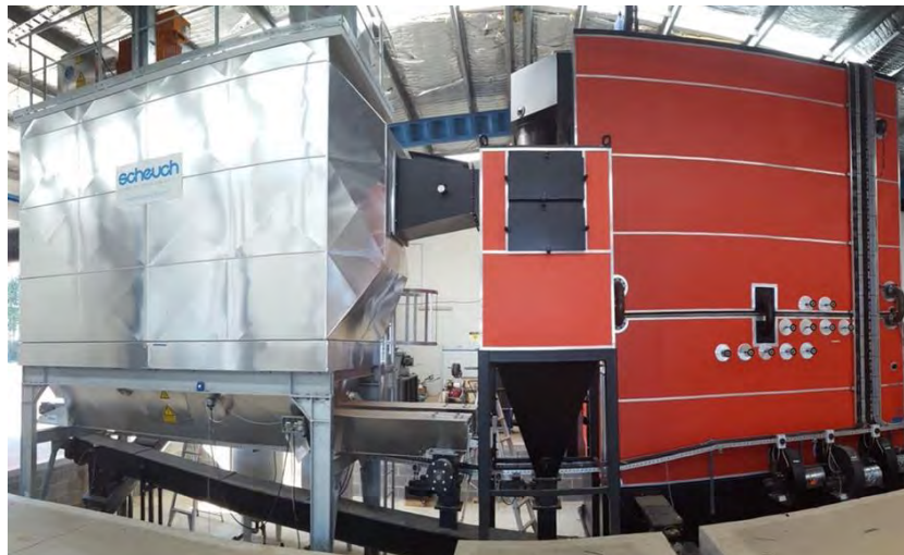
Figure 69: Biomass boiler (right) with exhaust gas treatment system (left). (Reproduced from Justsen Pacific.)
