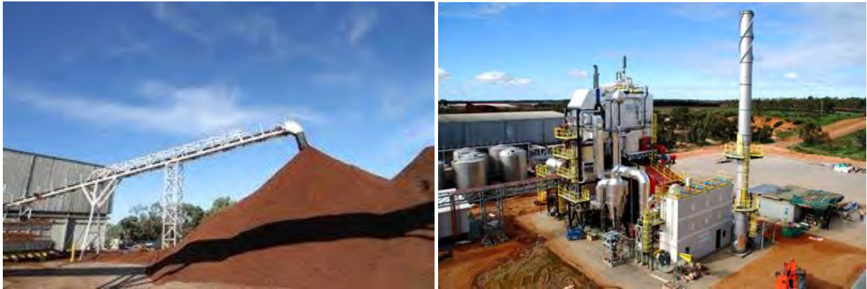
Figure 12: Automatic feed handling and 8 MW th boiler using grape marc. (Reproduced from Australian Tartaric Products.)
