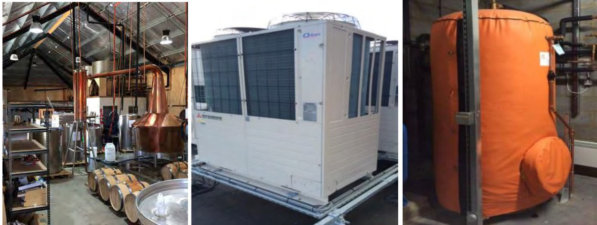
Figure 46: Left: Shene Estate and Distillery, TAS; Centre: Example of a Mitsubishi Q-ton unit; Right: hot water storage tank coupled to Q-ton unit. (Reproduced from Mitsubishi Heavy Industries).
