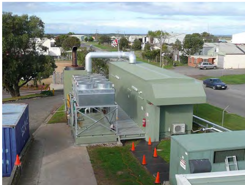
Figure 45: Midfield Meats Co-Generation system, Victoria. (image from Midfield Meats).
